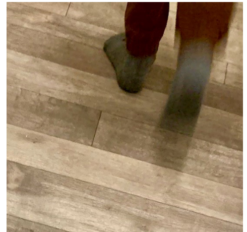
New floor installed in home to reduce asthma triggers.
